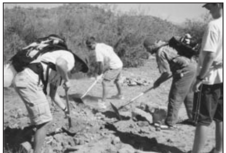
Trail Maintenance on Arizona Trail in Alamo Canyon.
