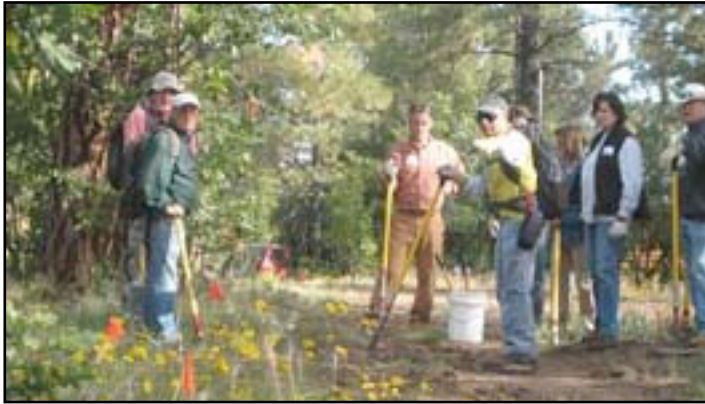
Crew Leader Richard Corbett outlines the day's work for the new Mormon Lake interpretive trail.
