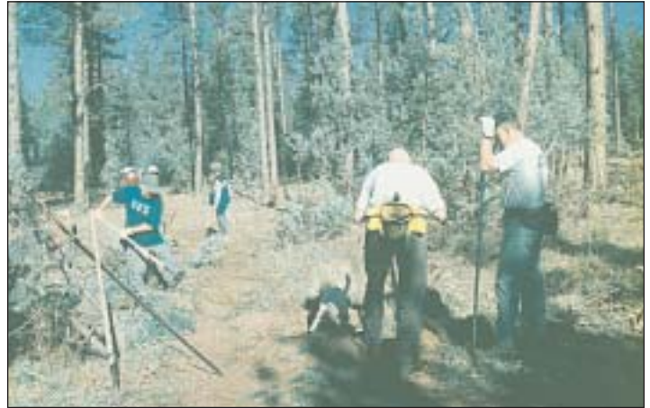
Gila County Trails Alliance crew working on Arizona Trail putting in signs and repairing tread.
