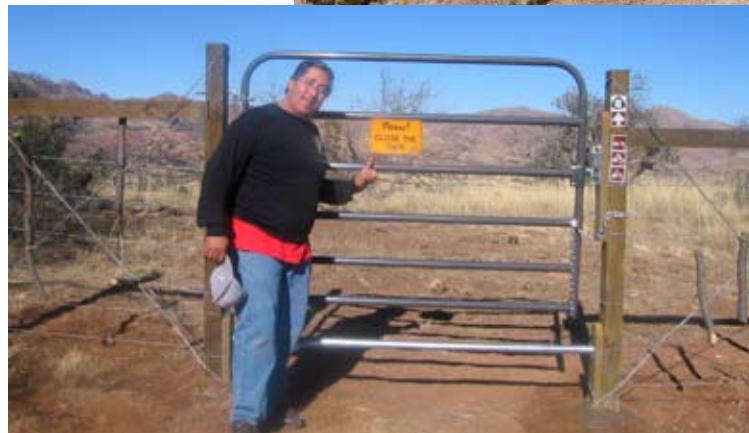
The first gate installed on the new Las Colinas segment of the AZT. George Lopez and Laddie Cox replaced the lag screw hinges with the more adjustable lag bolt hanger hinges, brought the concrete of both the latch and hinge posts to above the soil level, added the chain-snap-link latch, hung the "close the gate" sign, and added the decals. They then went on down the ridge to the north and worked with Bernie Stalman's crew building trail for an hour or so. Think of them when you "close the gate!"
