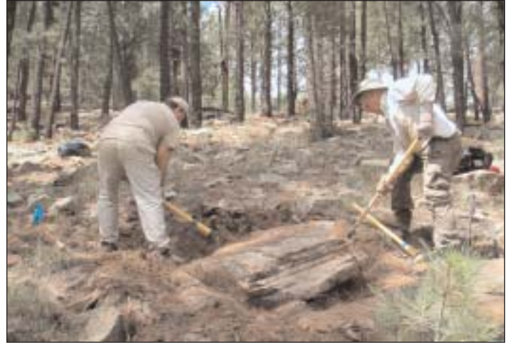
Big Rock - Rick Obermiller (left) and Laddie Cox tackle moving a big rock that had to go for the middle of the Trail route.
