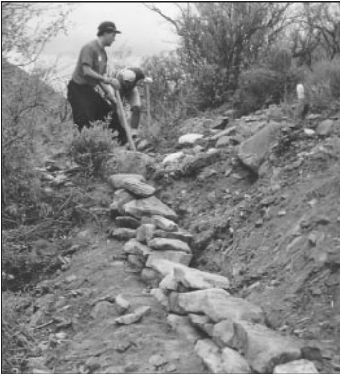
Building a section of Arizona Trail, Whitford Canyon REI Work Event.
