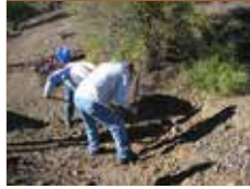
Working on the holes for the legs.
