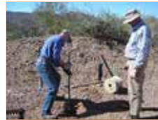
Finishing the hole manually.
