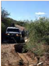
The winch sure beats trying to roll this with rock bars!
