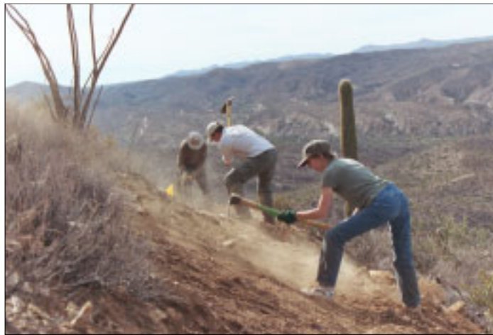
Trail workers will begin the challenging work of completing 25 miles of new trail construction in the Rincon Mountains when the project launches later this year.
