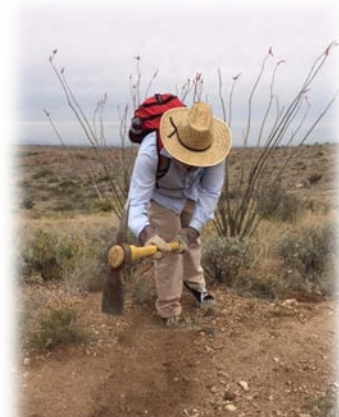
Digging a trench to help manage erosion.
