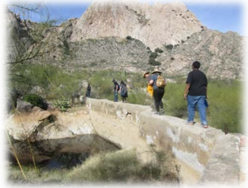
Crossing the dam, don't look down!
