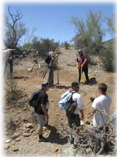
The McLeod crew working to create the new tread
